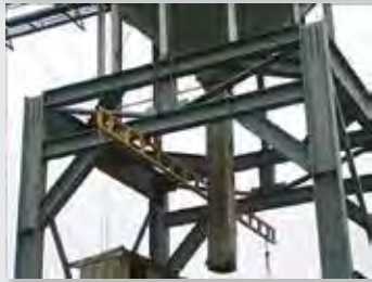
SPANCO Ceiling Mounted Fall Protection System mounted to a grain dispensing silo. System protects workers as they climb on top of rail cars to fill them with grain.
