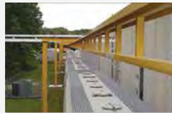
SPANCO Freestanding Fall Protection system with Long Span design. This particular system has 70' (21m) spans between supports. The system is used by workers who must access hatches on top of the rail cars.
