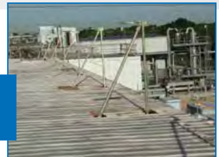
"StrongBack™" Rooftop Installation
